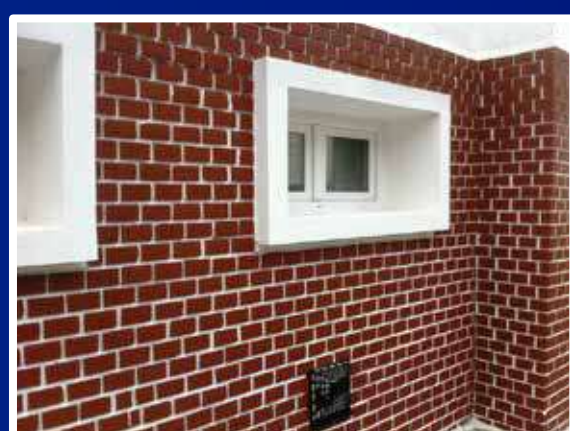
Clinker brick building
